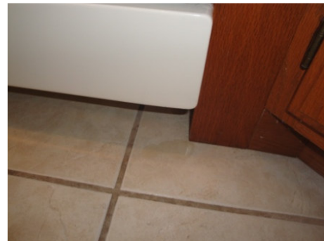
Figure 12: About a teaspoon of water under the dishwashing machine.
