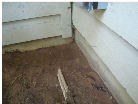
Figure 17: Low area next to the foundation.
