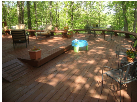
Figure 1: On the surface the deck appeared to be in good shape.
